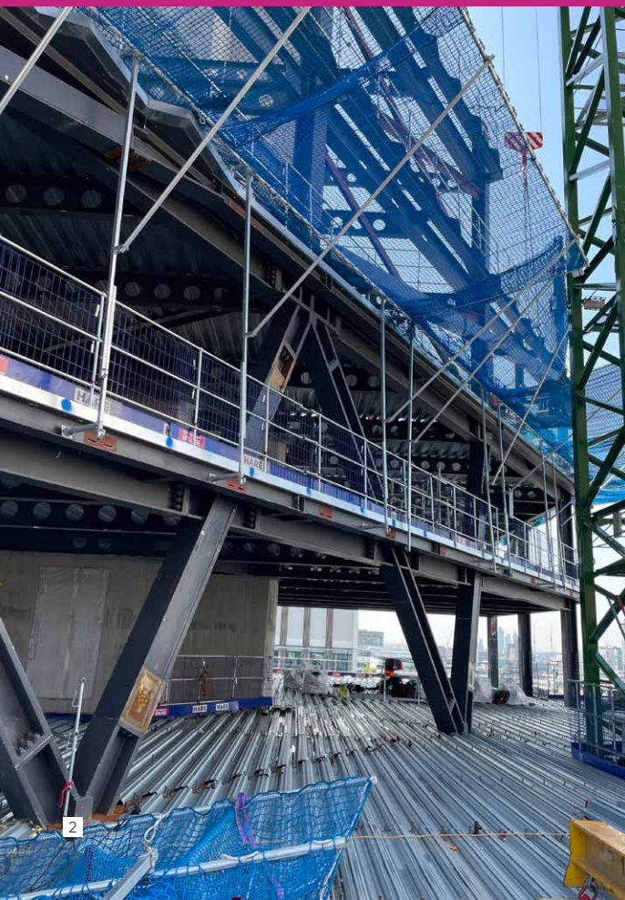
Figure 2: © ArcelorMittal, photo taken during job site visit in May 2025
